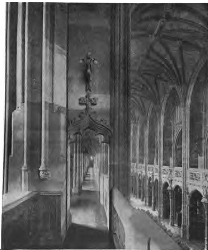
5. GALLERY CORRIDOR IN THE MAIN LIBRARY
